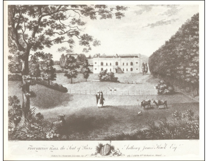
Stoughton Grange 1789, the residence of Major Powys-Keck in the early 1860s, from J. D. Bennett, Vanished Houses of Leicestershire, Leicester Museums, 1971. Although described by Throsby as Stoughton Hall, all other sources refer to the house as Stoughton Grange, which took its name from the original medieval estate (Reproduced by permission of Leicester Museums and Galleries.)
