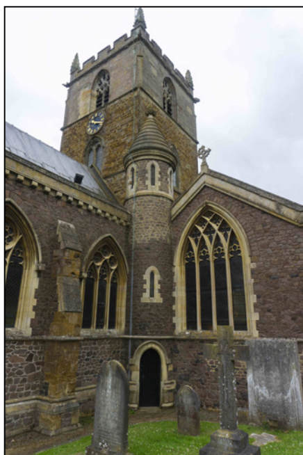
This small door at the base of the stair turret may have been the bell tower door at the centre of the 1862-63 dispute - but it may be of a later date when part of the church was rebuilt in the 1870s.
